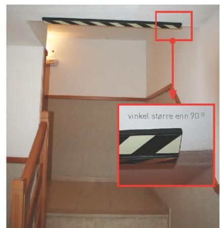
Støtdemper for flate overflater N 81 21
